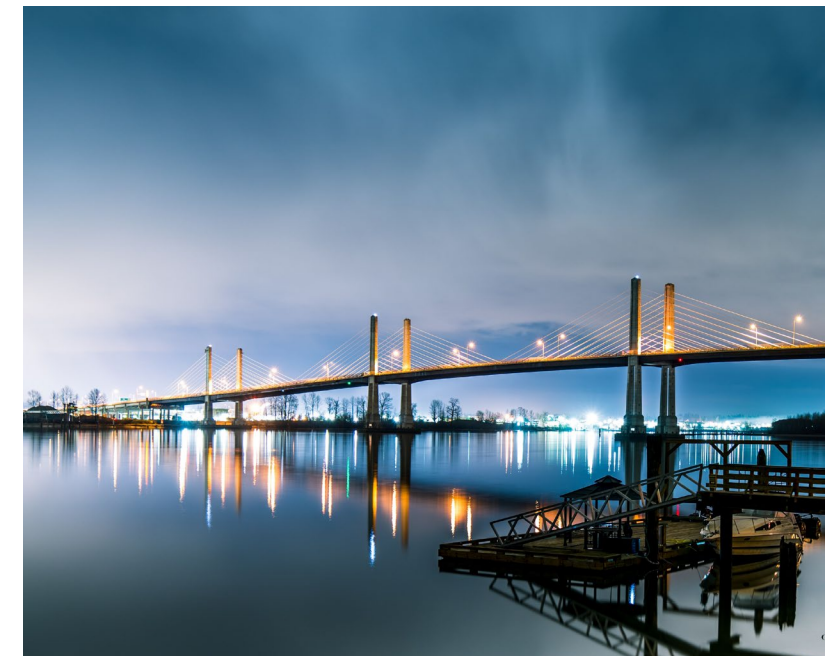
Golden Ears Bridge between Langley and Maple Ridge
