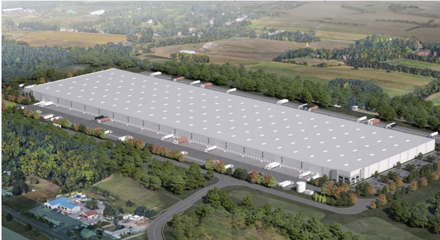
Prologis - 7600 Linglestown Rd, Harrisburg, PA
