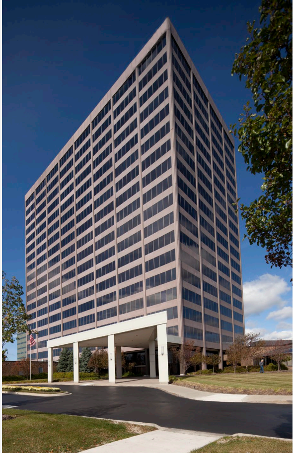
Travelers Tower I, Southfield, MI
