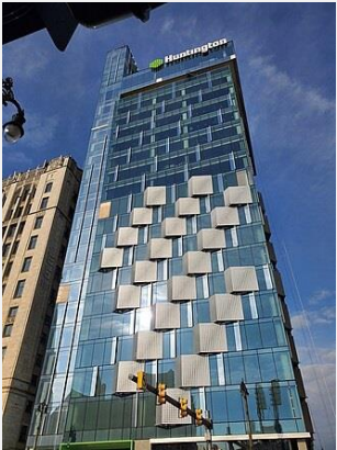
Huntington Tower, Detroit
